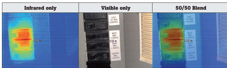
Figure 6. Equipment labels and the problem area can be read in an infrared and visible blended image
