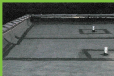
Cool areas on this roof exposure probably indicate moisture buildup. Mark with tape and investigate with core samples.
