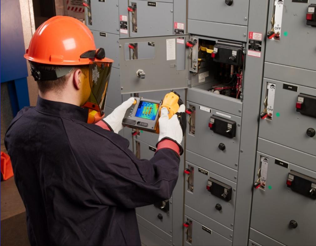
For troubleshooting, taking a thermal image of a malfunctioning unit can often identify the source of the problem—electrical hotspots can tell you which phase or connectors to check, motor hotspots can narrow it down to bearings, and so forth. Then, after repairs, follow up with another thermal image and verify that the component is no longer overheating—or that something else isn't now overheating, instead.
