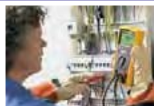
Insulation test at a distribution panel
